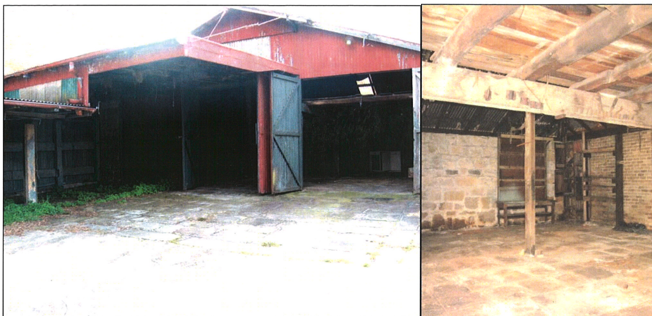
The stables/coach house at the rear of the Forsyth house 'Tyneside'
